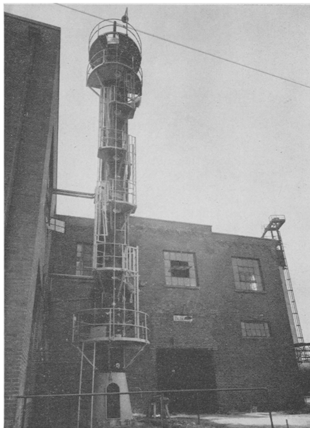
FIG. 3. The splitting column is about 60 feet high and is lined with corrosion resistant alloy.
